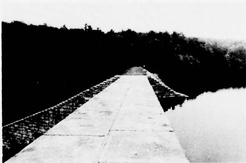
B. View Towards Right Abutment. Nonoverflow Section, Retaining Wall, and Embankment.
